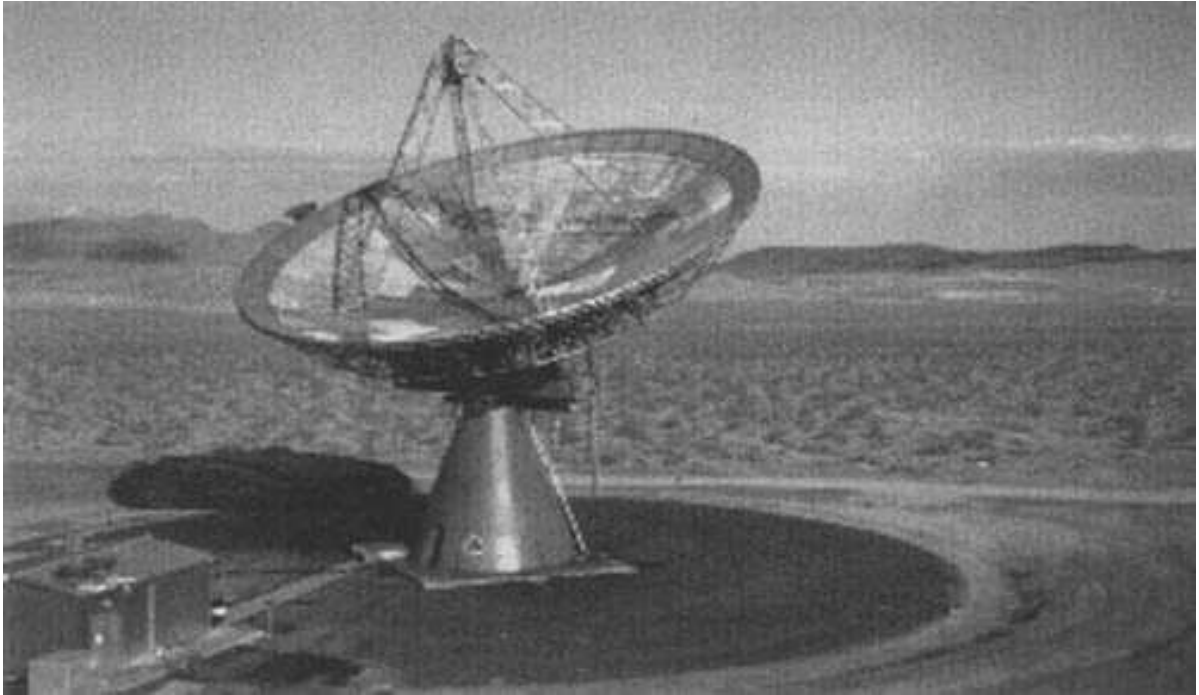
85 foot dish built for the Echo project by JPL at Goldstone Dry Lake
